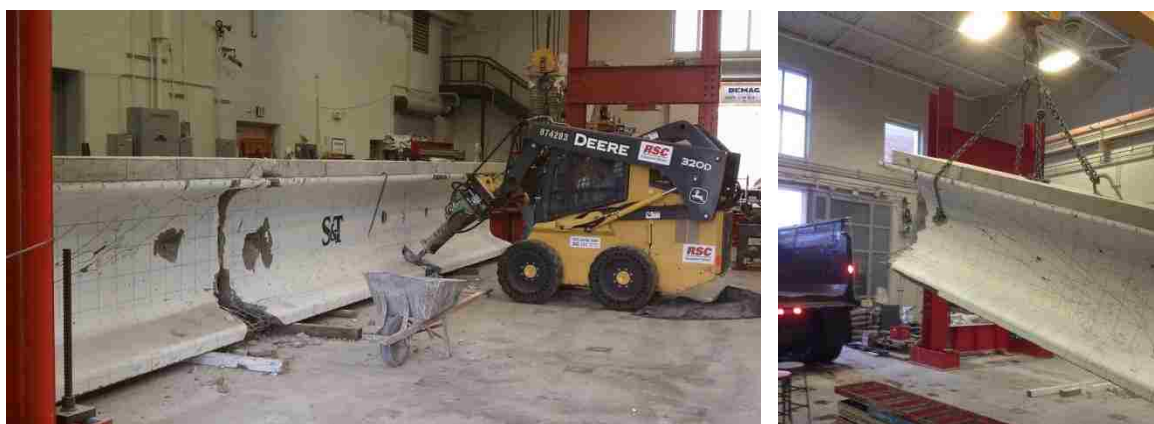
a) Demolition of Test Girder
