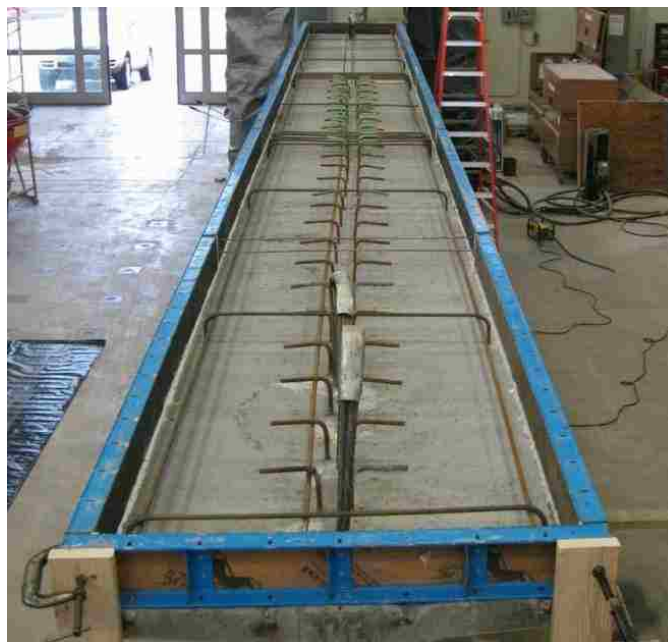
Figure 3.13. CIP Deck Preparation
