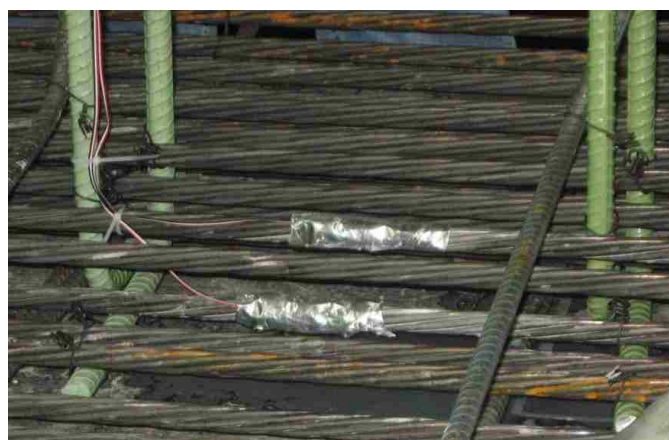
Figure 3.7. Strain Gauge Installation
