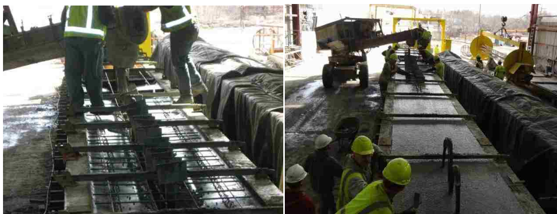
Figure 3.8. Fabrication of Test Girders
